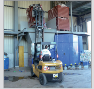
Filling by means of a lift truck
